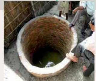
Pits smaller than required
