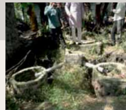
Pits smaller than required
