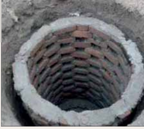
Excessive honeycombing
